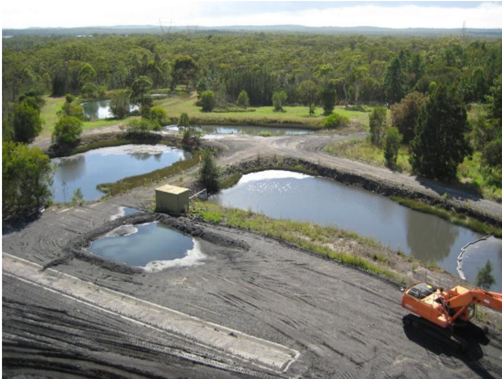
Plate 7.21: Pond B water management control system
