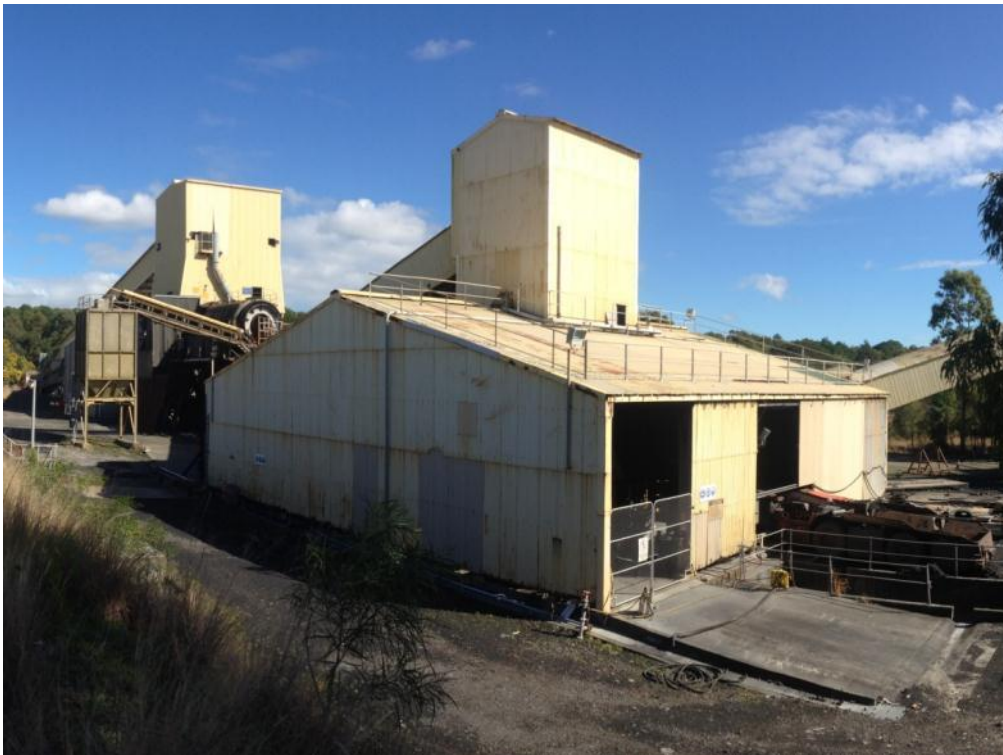
Plate 7.4: Mannering coal clearance and processing facilities
