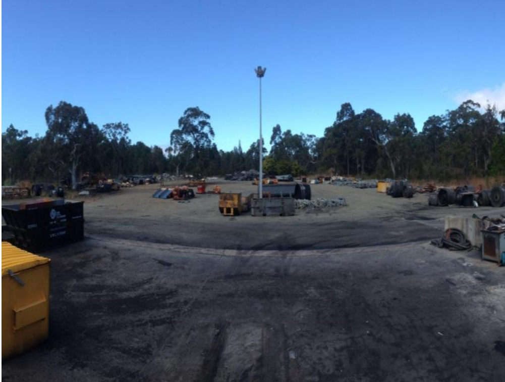
Plate 7.5: Mannering hardstand (eastern storage area)
