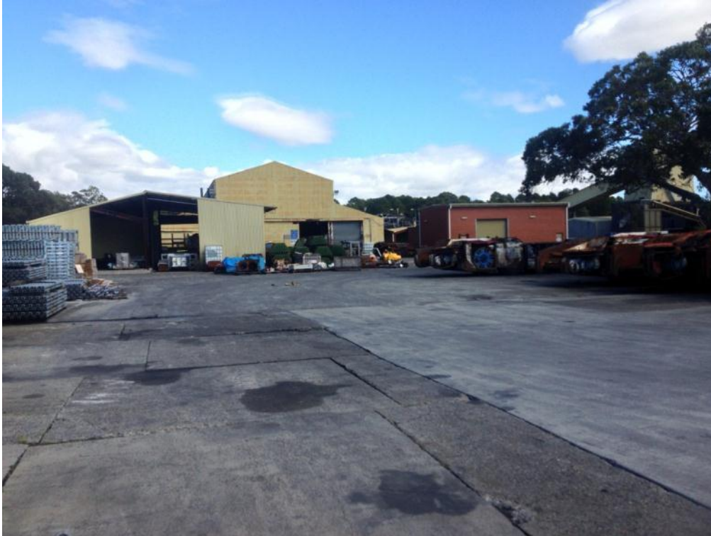
Plate 7.3: Mannering hardstand area
