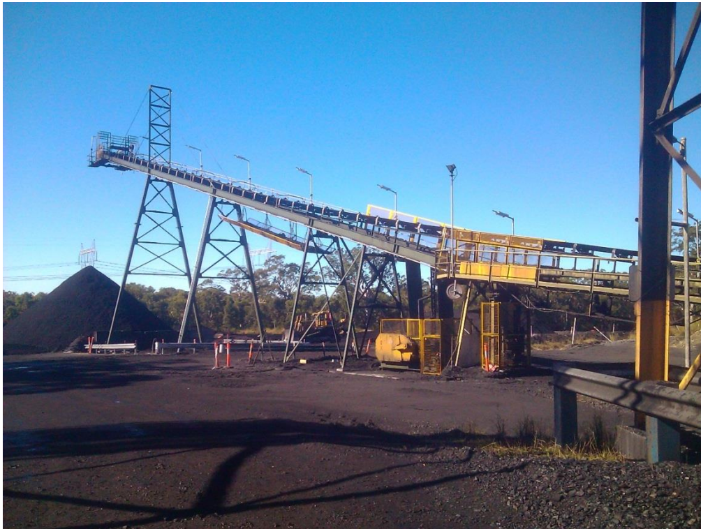
Plate 7.20: Chain Valley stacker conveyor
